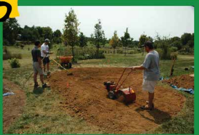
Dig, add soil modifications, mix soil & level*
