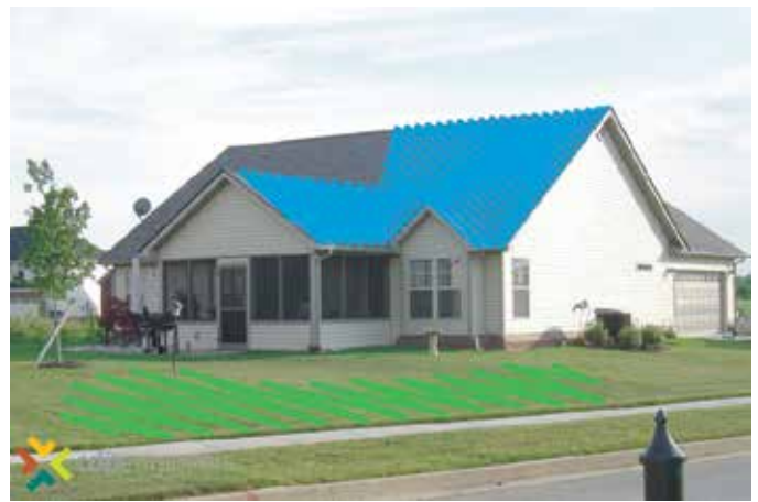
This rain garden (seen above) is designed to capture water from the highlighted portion of the roof based on the downspout configuration and rain garden location.
